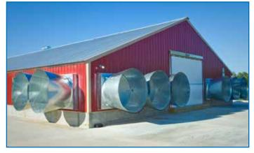
The system uses fans (usually 122 cm [48 in] or 127 cm [50 in]) at one end of the house, and air inlets at the other end. High volumes of air are drawn down the length of the house, exchanging the air in the house in a short time (**Figure 111**).
